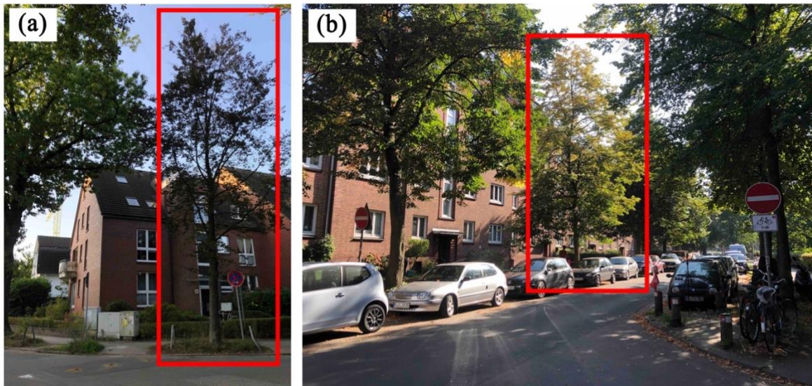
Figure S8 - Example of unhealthy trees (red box) affected by a gas leaks in close vicinity, HH004 (a) and HH010 (b)
