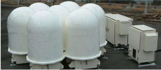
Figure 1. WPR LQ-7 Luneberg Lens antenna array.
