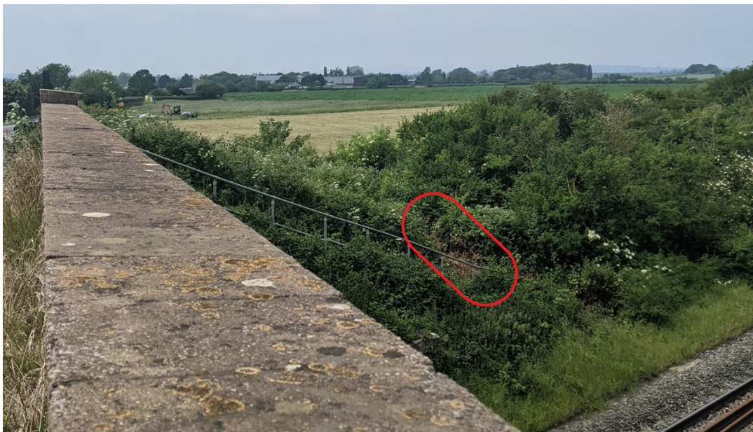
Figure S2. Image of dead vegetation (circled in red) at gas leak site taken on 12 th June 2023.
