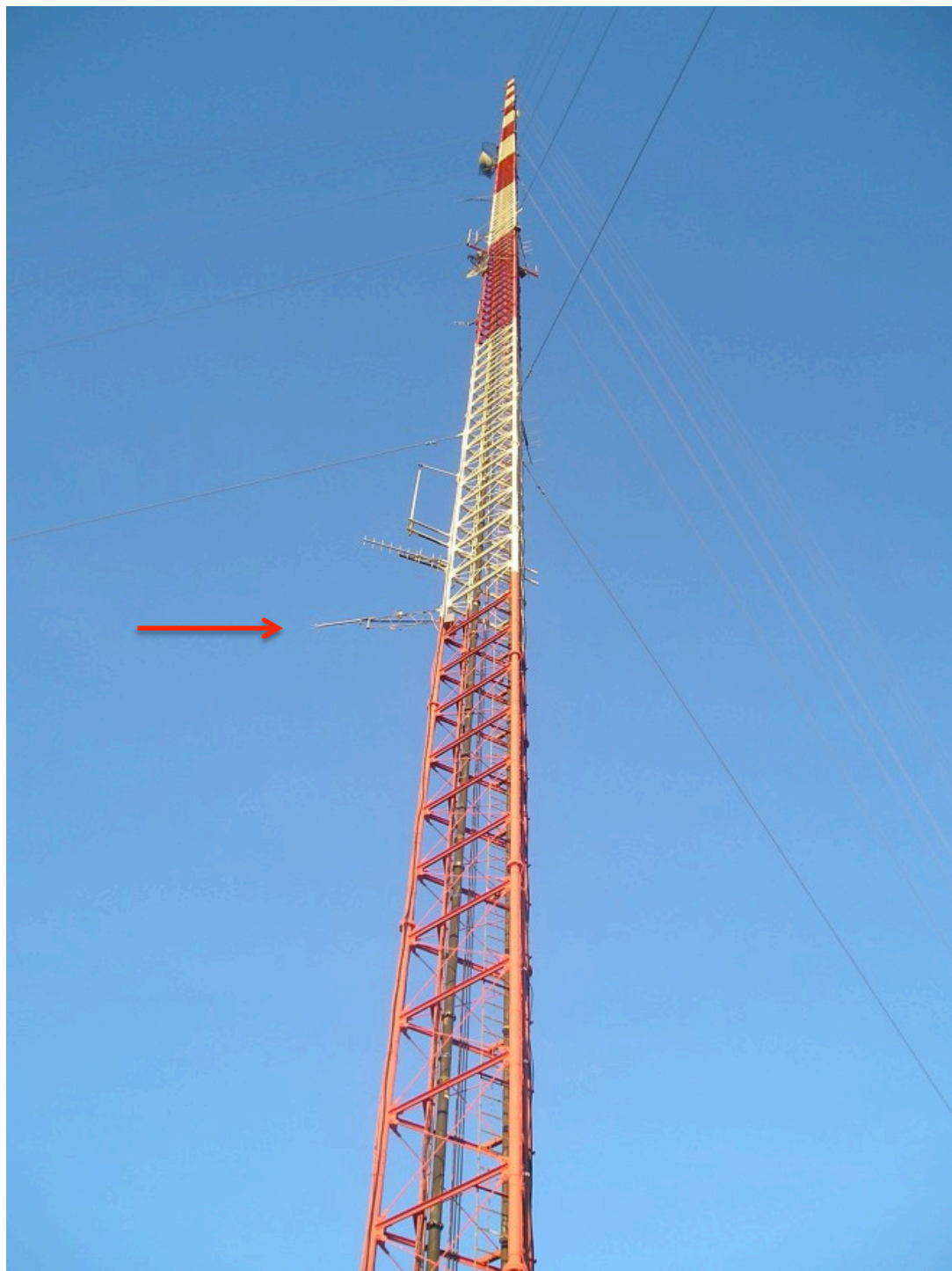
Figure S1. WLEF-TV transmitter tower near Park Falls, WI, which is the NOAA site LEF. Booms with meteorological sensors and gas sampling inlets are installed at 30, 122, and 396 m. The 30 m boom is marked with a red arrow.
