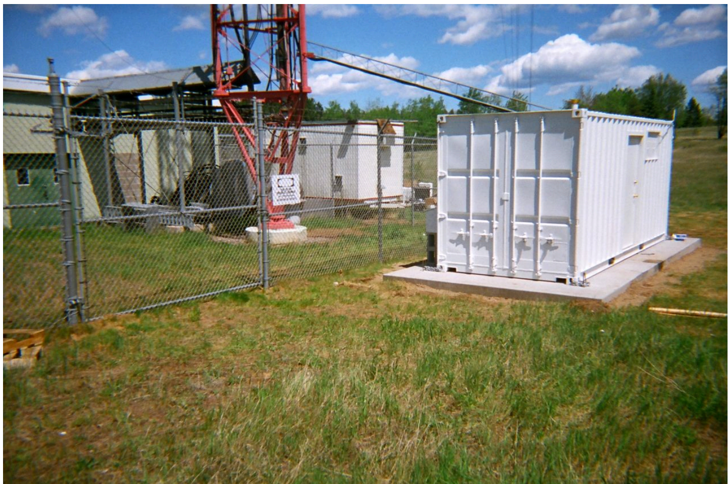
Figure S2. Sea container laboratory installed at the base of the tower at LEF. Large doors on the end of the container facilitate installation of equipment.
