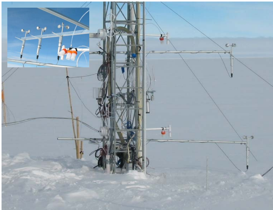
Fig. 1. Photograph showing the setup of the ozone flux gradient experiment on the Summit flux tower. The picture depicts the two lowest measurement heights (2 m, 0.75 m) only. Instruments are pointing towards the south, the dominating wind direction at Summit. Each gradient height measurement consists of a wind speed measurement (located furthest to the right in the picture, supported by the cross arm, a temperature measurement, with a downwards pointing inlet from the aspirator, and an ozone inlet funnel (in orange). The insert in the upper left corner shows the cup anemometer and ozone inlet arrangement during an inter-comparison experiment.
