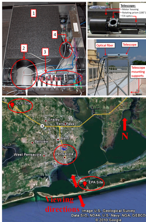
Fig. 1. Figure 1: updated so the inside of the rack can more easily be seen - additionally the caption has been appropriately modified
