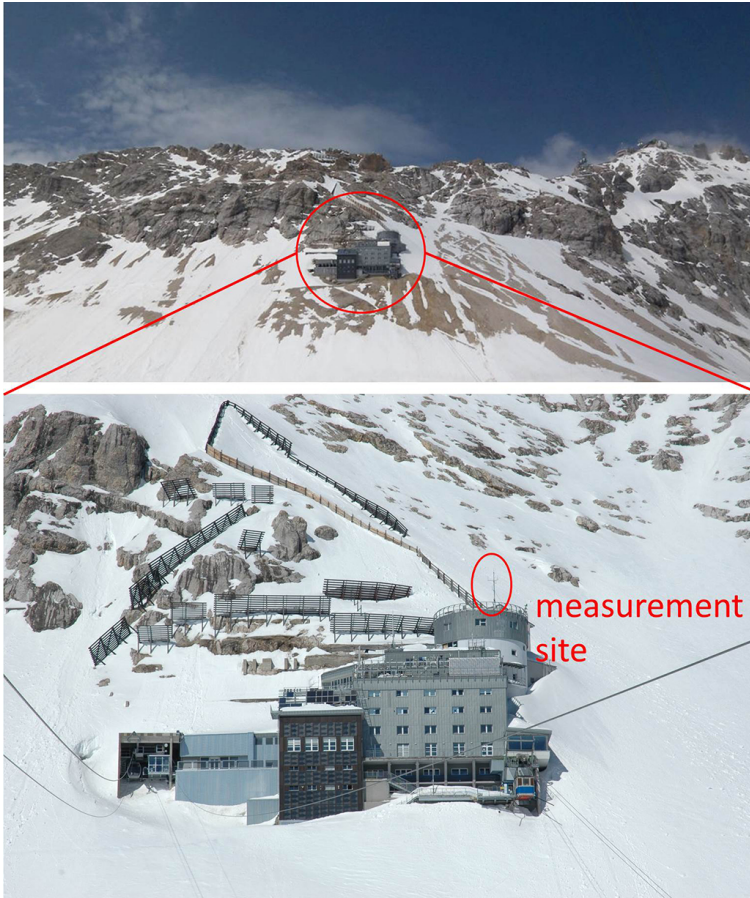
Figure 1. Views of UFS from the south. The lower picture is a close-up view of the top picture and the measurement site is indicated by the red ellipse.
