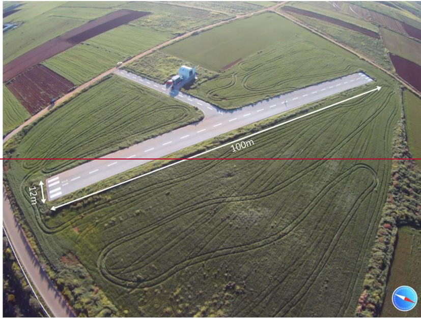
Figure 2: Aerial view of the Grounda runway in Cyprus.
