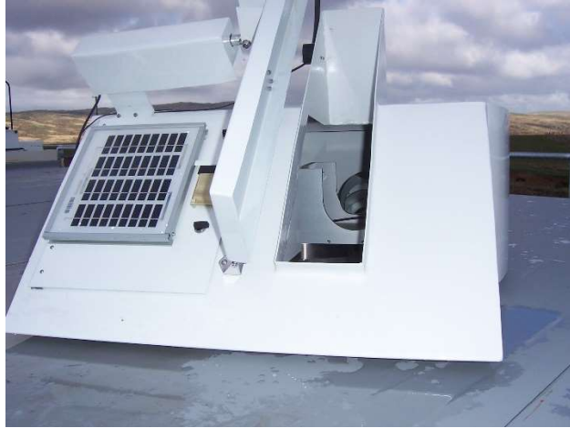
Figure 14: Our completed tracker inside matching automated weatherproof cover
