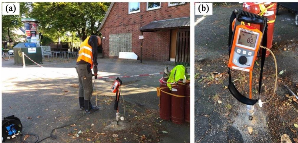
Figure S3 - Drilling holes around the surface-projected track of gas pipeline (a) and measuring the \text{CH}_4 mole percentage (b) to find the gas leak location, HH008
