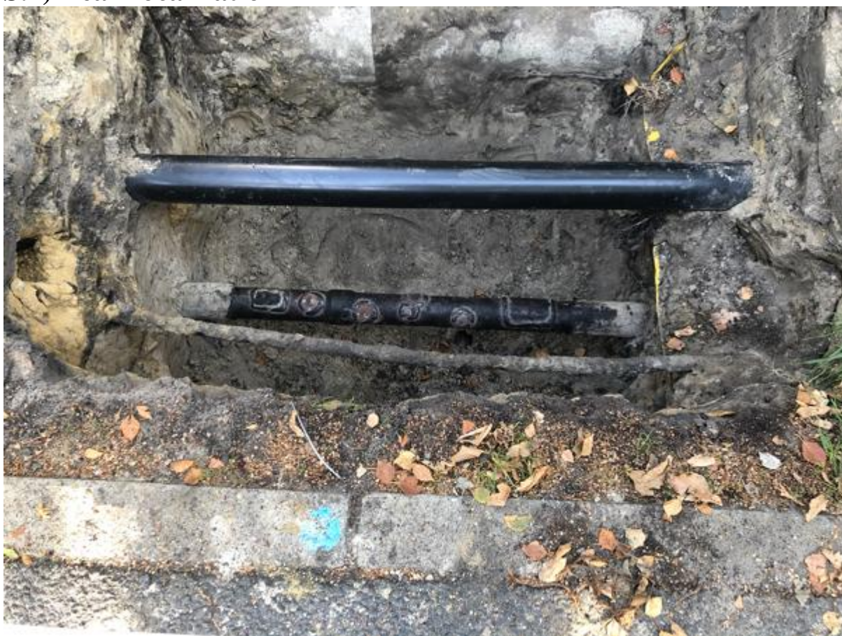
Figure S9 - The LDC reported 6 leaks on the pipeline at this location with total leak area of 5 cm 2 , HH013
