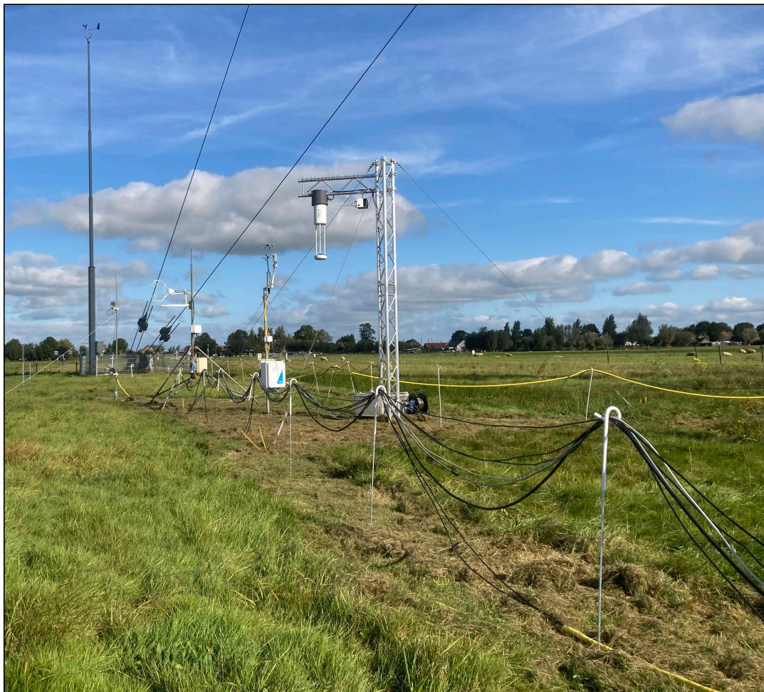
Figure 2. The instruments, seen from the miniDOAS container looking north. From left to right: 10 m wind vane mast, mast with the two retroreflectors of the miniDOAS instruments, mast with sonic#3, mast with sonic#1 and LI-7500DS; mast with HT8700E and its cooling unit. Sonic#2 was placed later at 40 cm on the southeast side of HT8700E on the same mast (not shown in the photo). The 213 m mast is off to the right (east).
