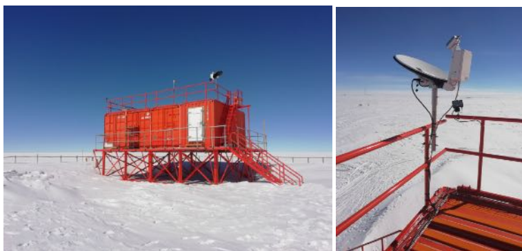
Figure 2. Left side: PHYSICS shelter at Concordia station. Right side: Micro Rain Radar (MRR) installed in 2018 on the roof of the shelter.
