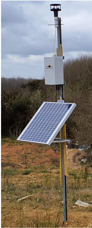
Figure 1: System A autonomous field logger (LSCE007) installed at the SUEZ Amailloux landfill site in March 2021 (see text for description). This system includes a two-dimensional anemometer.
