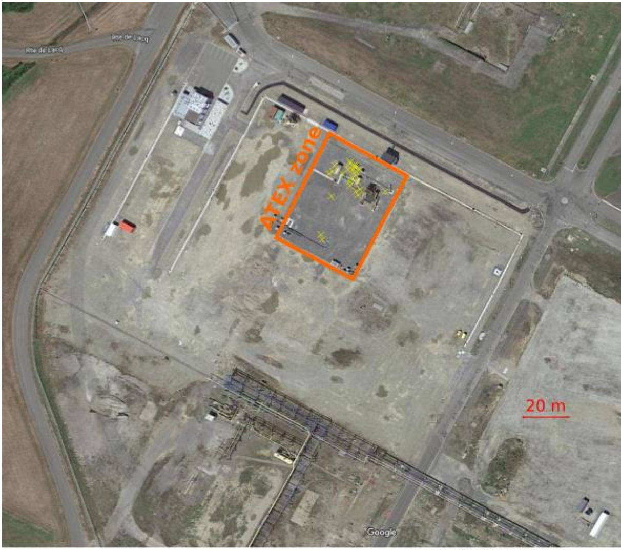
920 Figure 5. Aerial view of the TADI platform with location of the emission sources (yellow crosses) and the Explosive Atmosphere area (ATEX zone, depicted as an orange square). Maps Data: Google, ©2022 Maxar Technologies.
