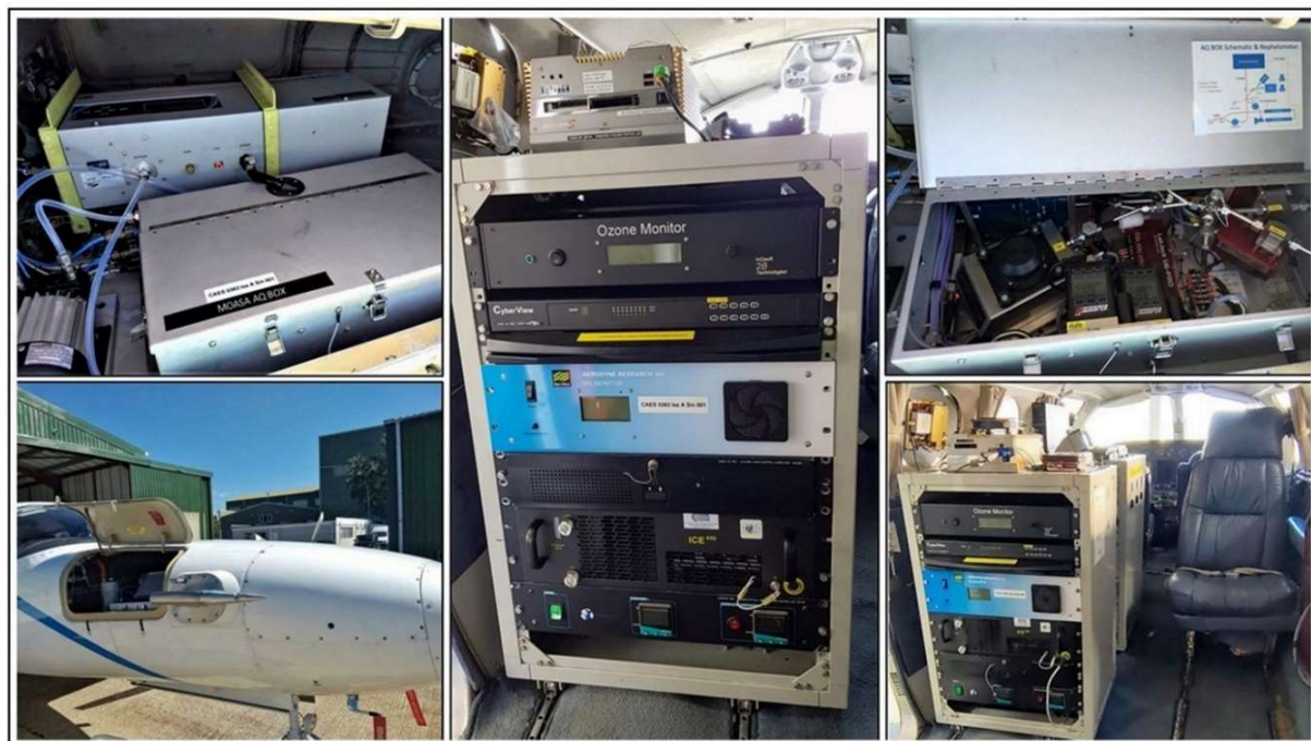
Figure 2: Clockwise starting top left: the AQ box (foreground) and nephelometer (background) in the MOASA nose bay; the aft instrumented rack housing the O 3 , NO 2 and aerosol LIDAR control system; inside the AQ box; inside the cabin looking forward; the Brechtel isokinetic air sample inlet and nose bay of the MOASA.
