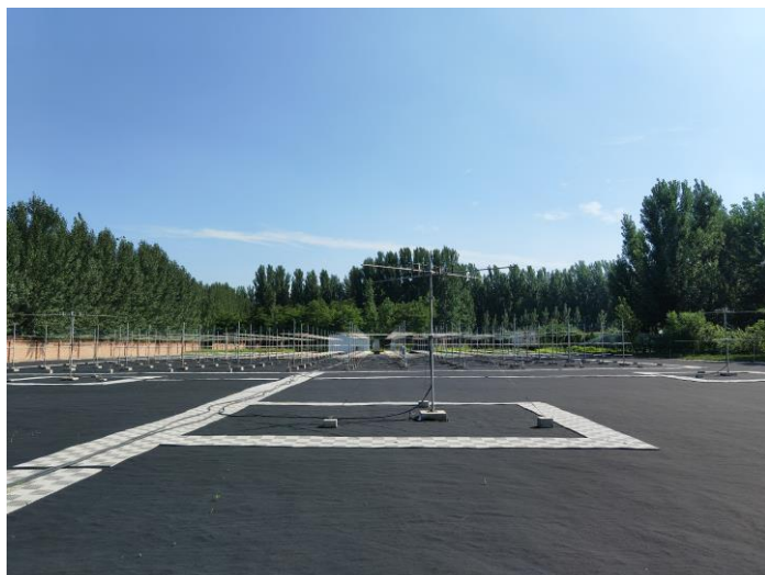
(a) Outdoor antennas
