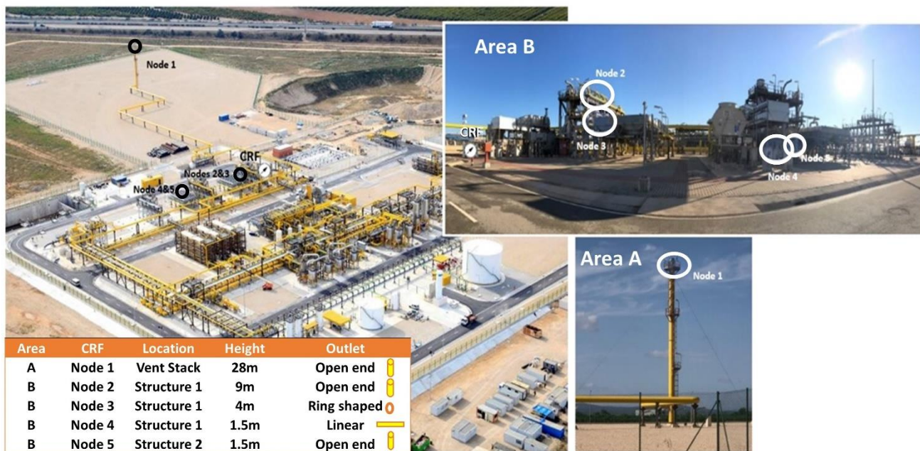
Figure 1: Aerial view of the Enagas site in Spain and node location (white circles). The controlled release facility is indicated by a white disk marked “CRF”.
