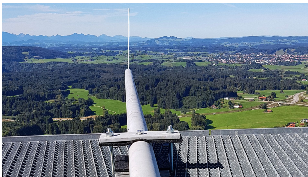
Figure 2. Horizontal LPR installed at 245° AZ at the Radar MOHP during the measurement campaign.
